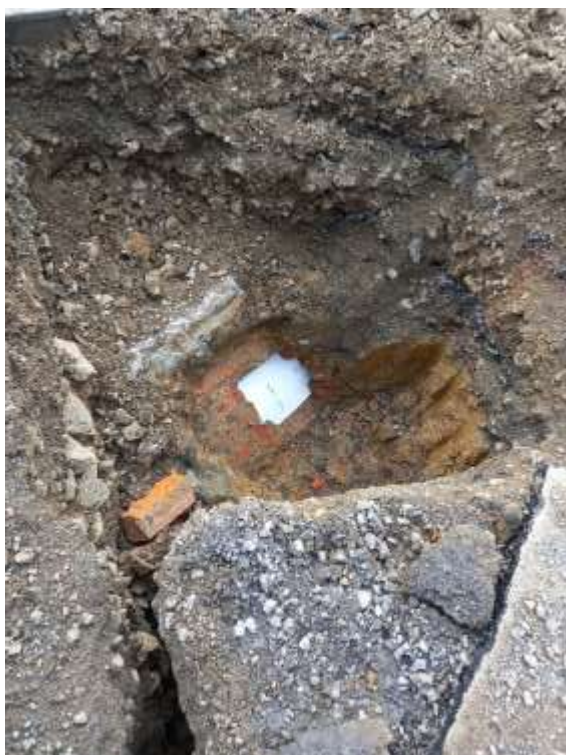
Brick barrel drain Nick Morris, LT McGuinness
