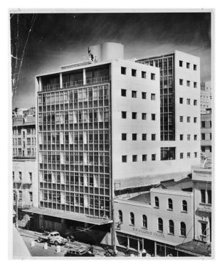
Although now a common feature, at the time of its construction the large expanses of glass were striking against the heavy masonry of its neighbours. Unlike them, Massey House's structural system meant the front facade did not need to help carry the building's load, so a glass curtain wall was possible.
