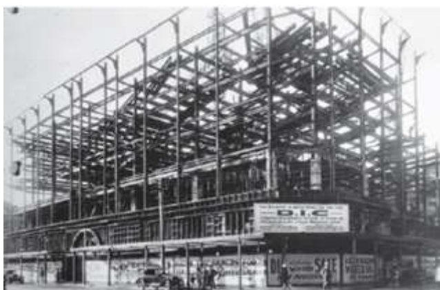
Steel framed construction of the DIC building, Lambton Quay, 1928 and its completed state in 2021 (Images: Richard Norman)
